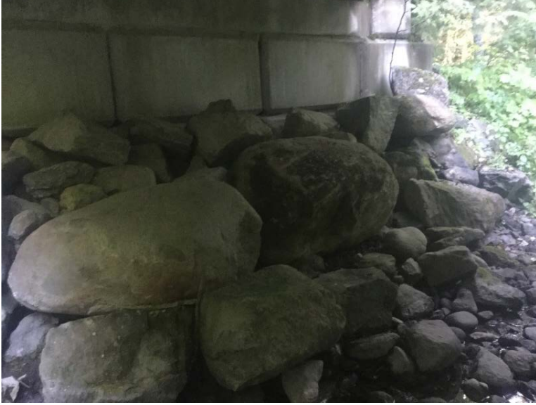
Left Bank Abutment when facing downstream
