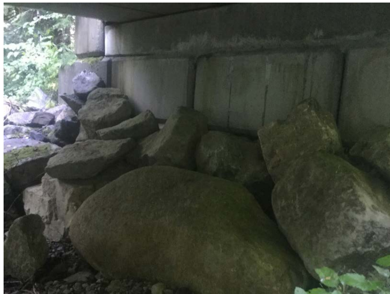
Right Bank Abutment when facing downstream
